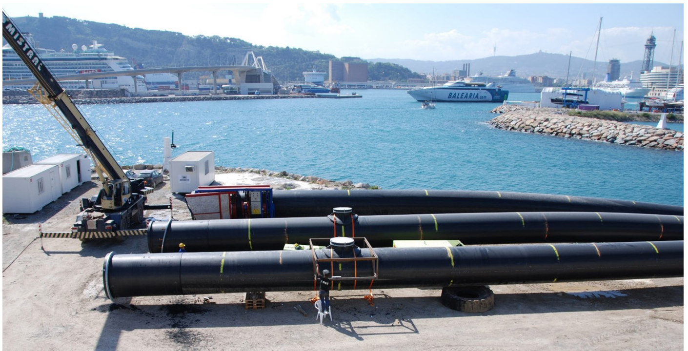
Pipe preparation for stub-end welding prior to delivery (Tangiers) and manhole installation (Barcelona)
