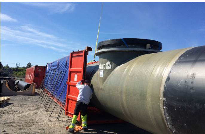
OD2000 mm T-piece with reinforcement
