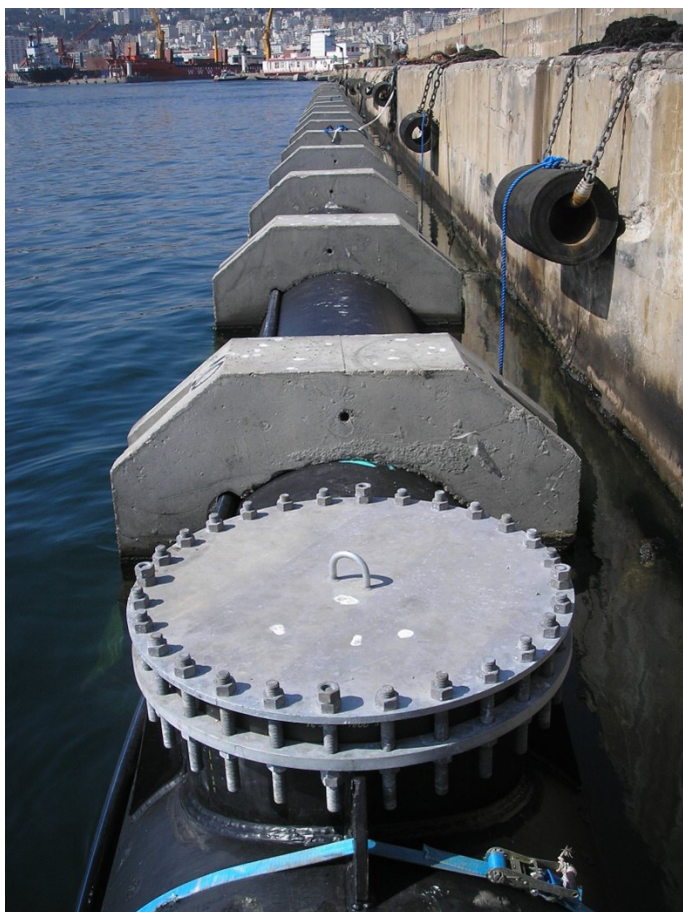
Completed saddle fitting with temporary blank flange
