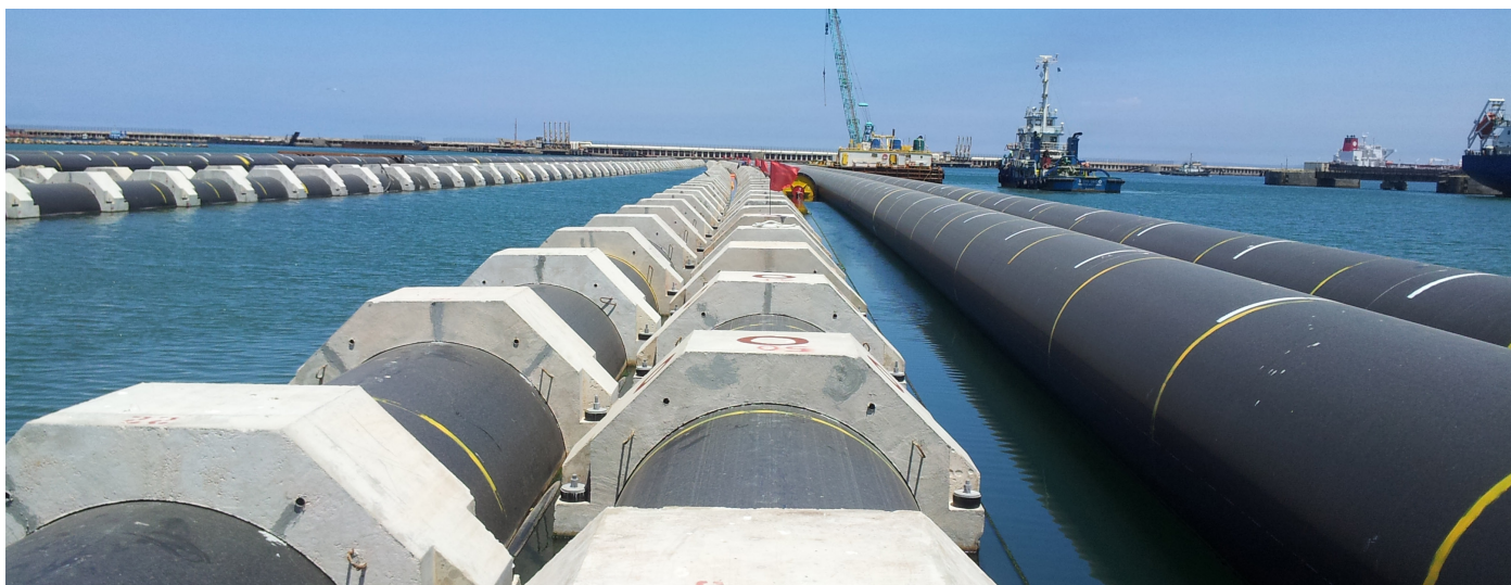
Typical pipe collar weighting for marine installation
