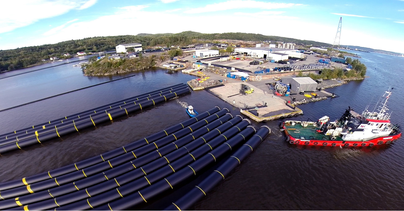
Pipelife Norge Stathelle plant
